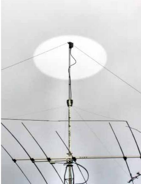
PHOTO 2: 80m dipole over the top of a small HF beam.
